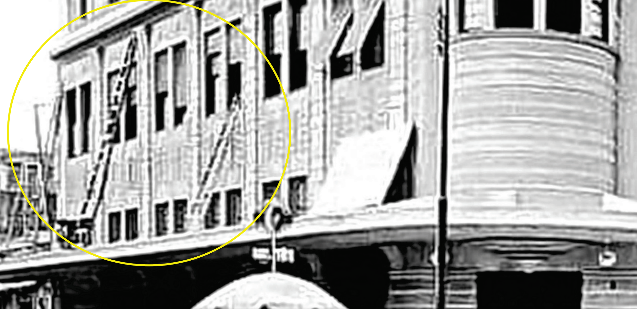
The building appears to be in the process of construction or repair, perhaps due to the earthquakes in 1917-1918 (Guatemala del Ayer, 2012).
