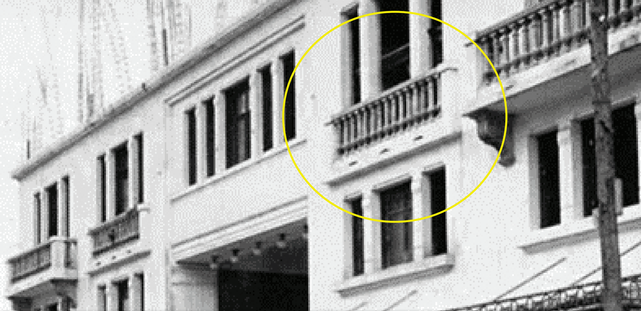
The architectural style represented is Art Deco. It is characterized clearly by the design of the white banisters on the second floor ...
