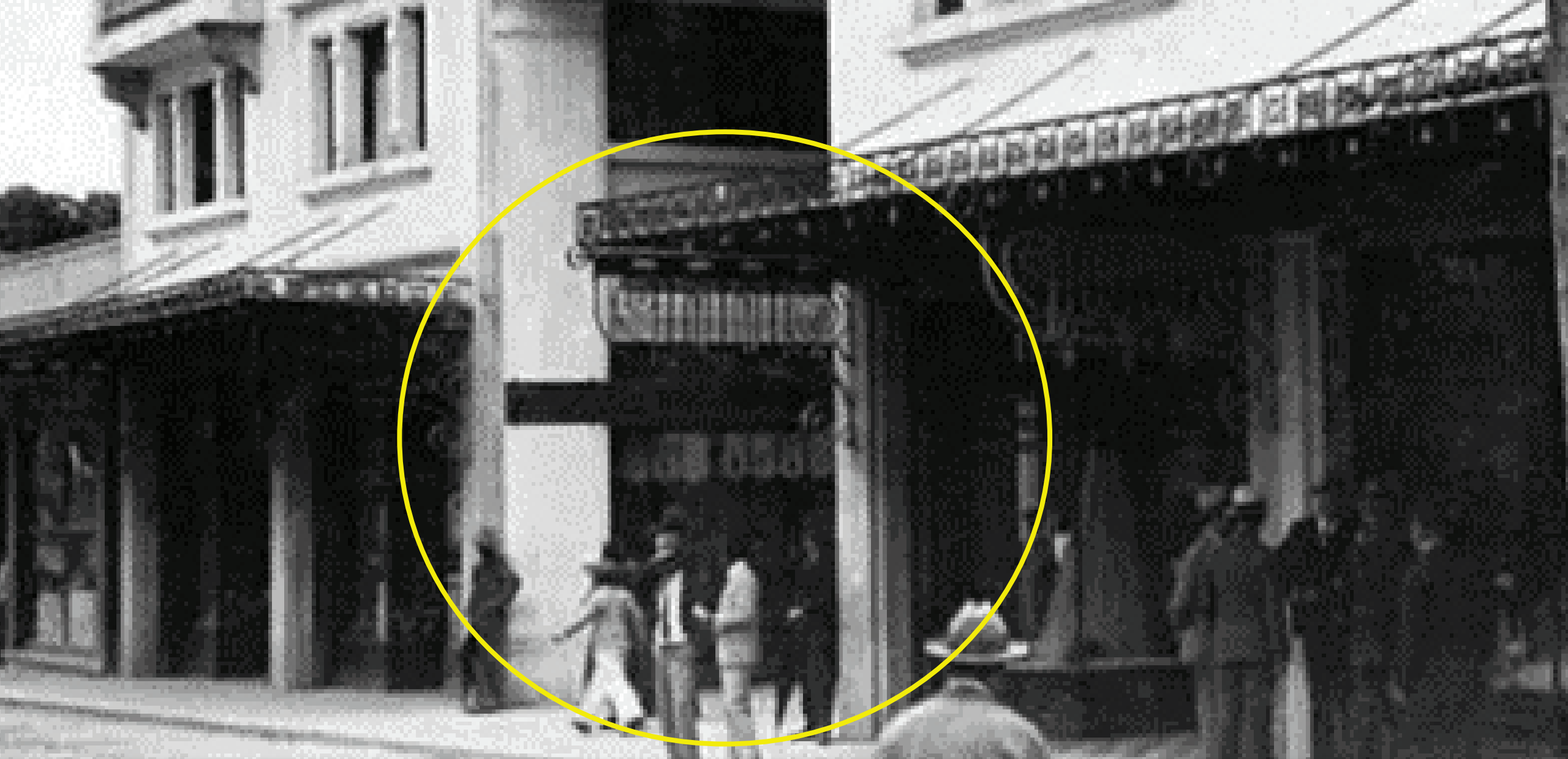
To the left of the display there is a large opening. It is the entrance to Pasaje Rubio. It also includes a large decorated wrought iron gate, perhaps intentionally used for fashion and/or security.
