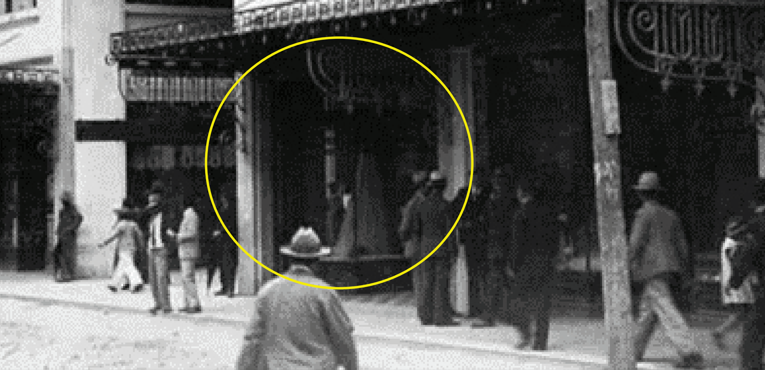
Below the iron awnings there is a store display.
