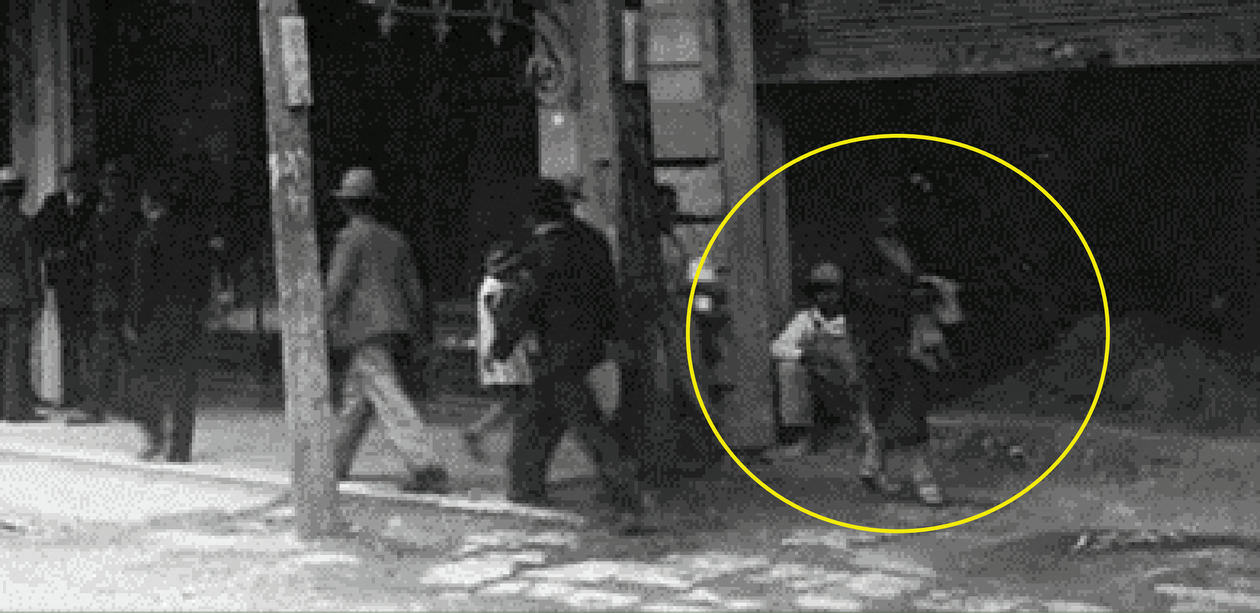
An individual with a black dress walks by in front. She has a face covering and is holding onto a smaller looking clothing item, maybe a sweater or jacket. The construction worker is directing his gaze towards her.
