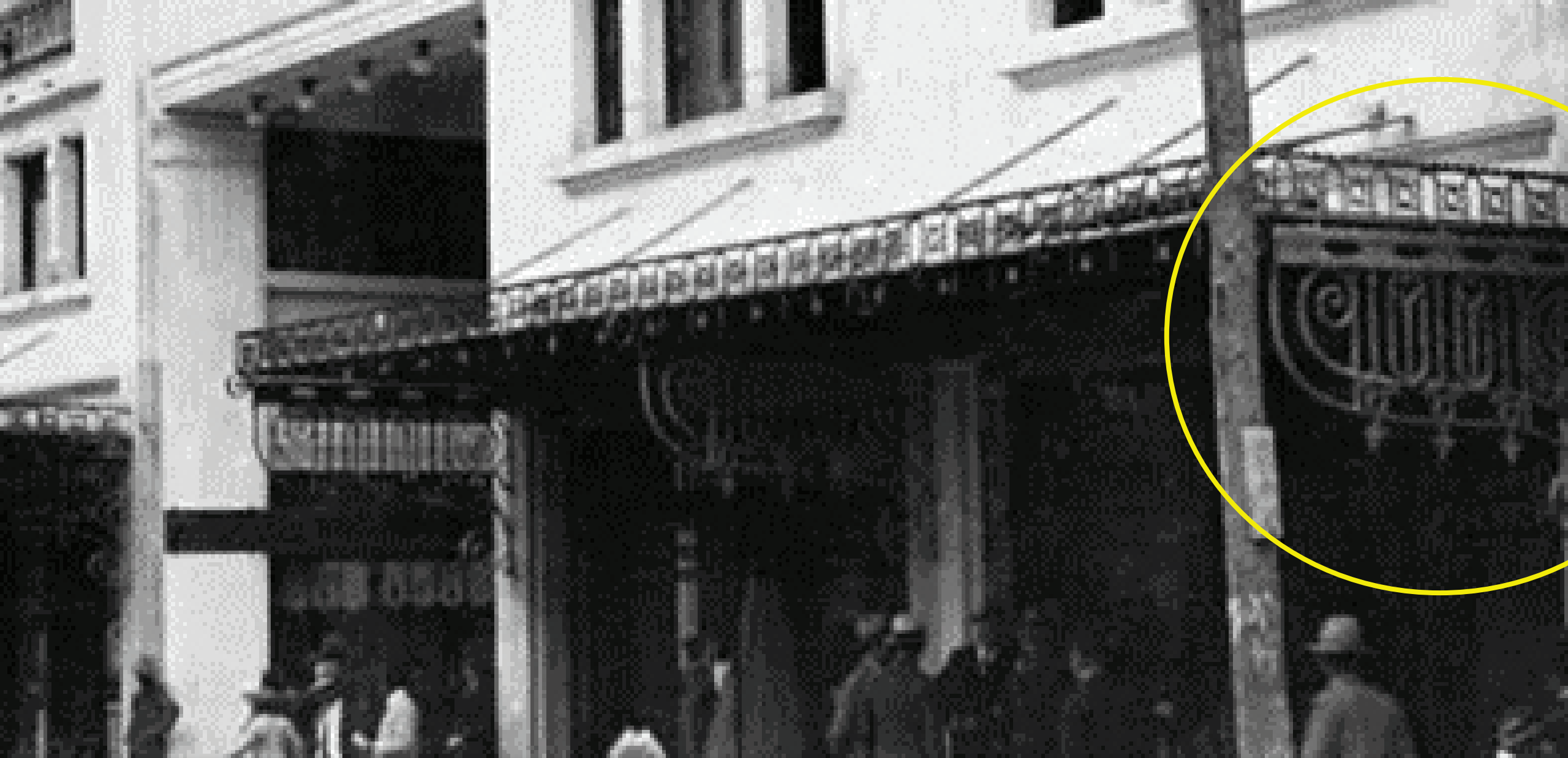
... and iron awnings on the first floor.
