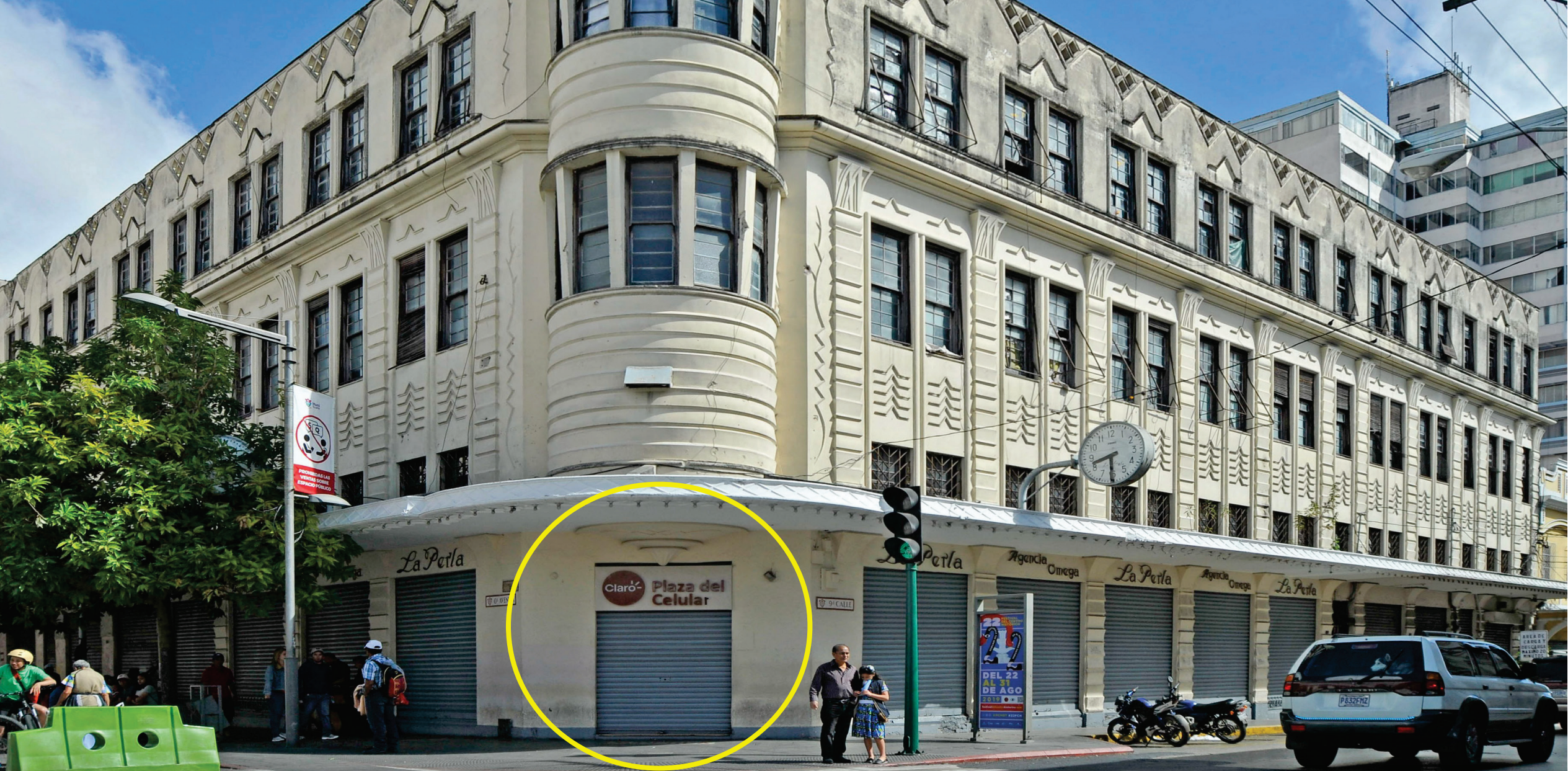
Today, the first floor is no longer a jewelry store but now houses various businesses, such as the cellphone conglomerate Claro. The first-floor storefront displays are now reinforced by steel gates. This is part of general security measures for businesses across the country during their non-operational hours.
